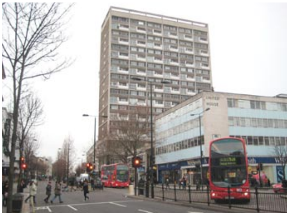
The Pears Group - Campden Hill Towers and north side commercial properties
