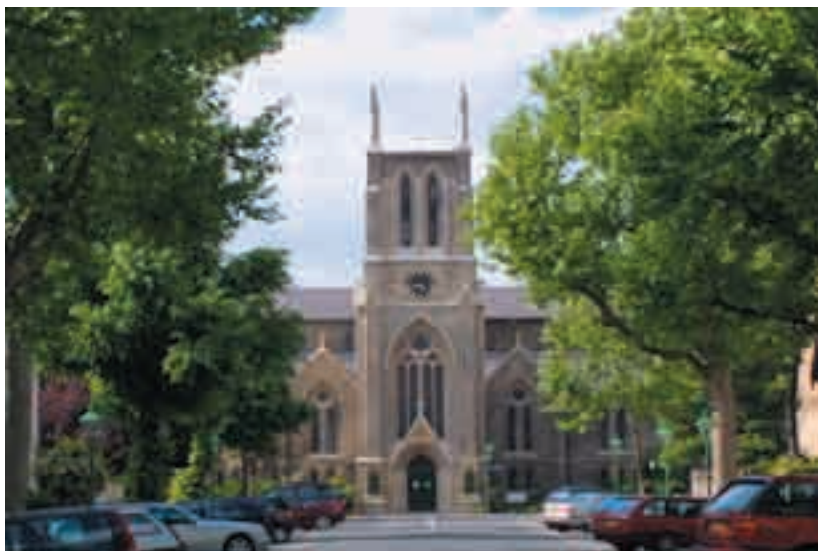
The photograph shows St. James's Norlands Church in Addison Avenue. (See inside for comment on the proposed mobile phone aerial).
