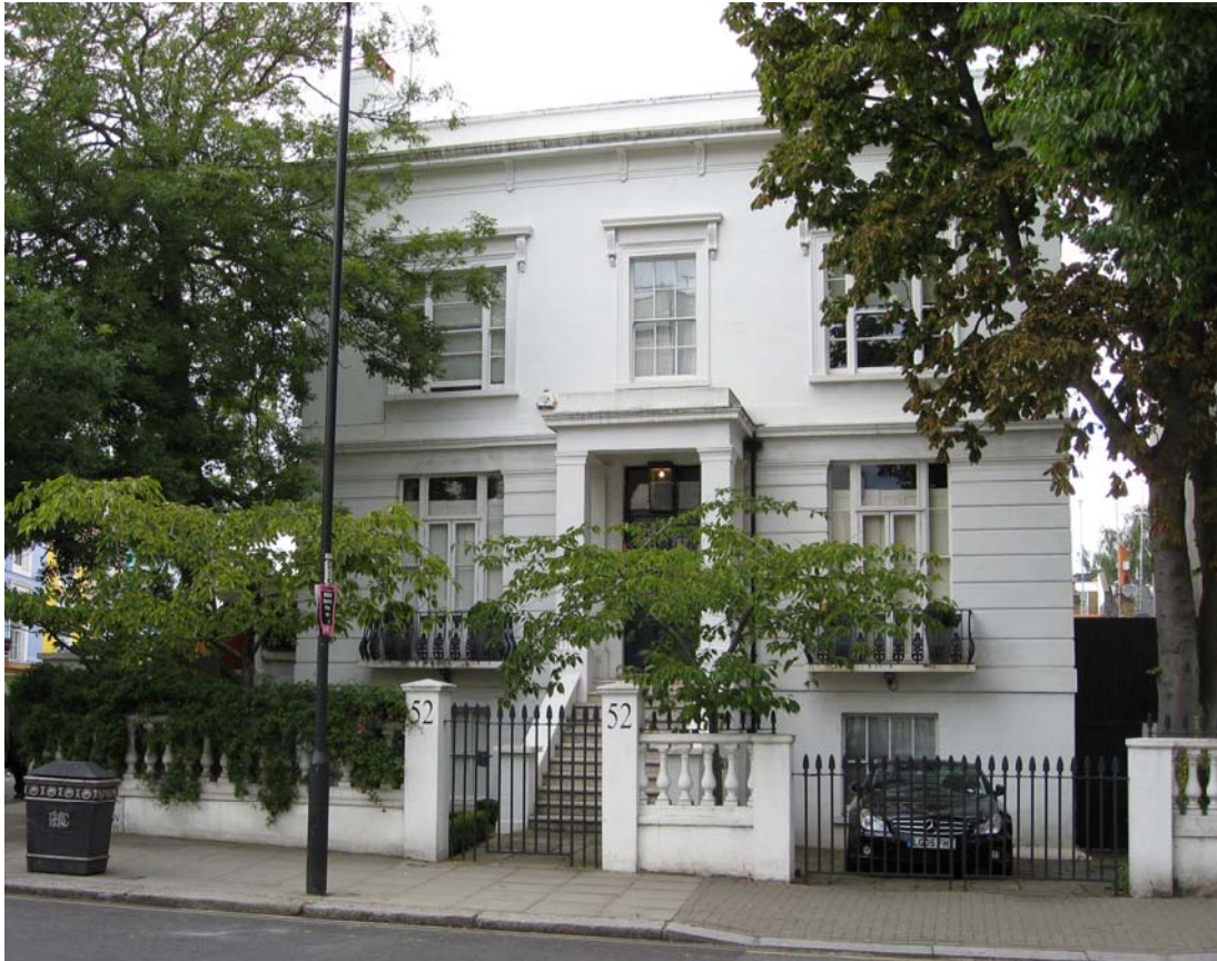
52 Chepstow Villas. In the 19 th century it was the home of a great-nephew of Napoleon, and in the 20 th century was the childhood home of the novelist Monica Dickens (see below). ( Photograph 2008. )
