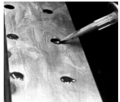
ill. 8: Pouring of screw holes
